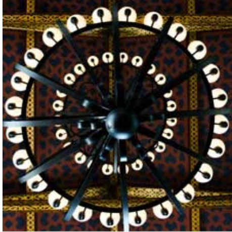
Figure 2. LED bulbs in this difficult to reach chandelier have not needed to be replaced in over a year. Previous generation bulbs burned out within two months [5].
